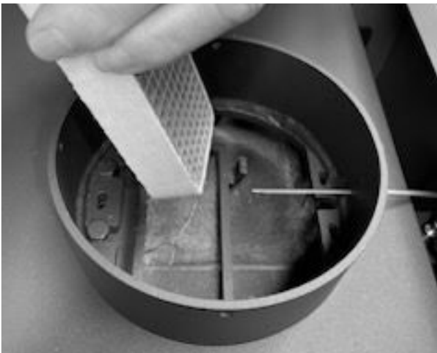
Figure 2: Insert combustor into flue.
