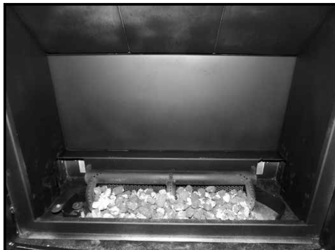
Figure 46: Burner basket with embers.
