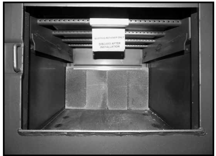
Figure 20: Bricks against rear wall.
